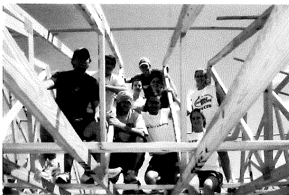
Habitat for Humanity work crew, Miami, FL
